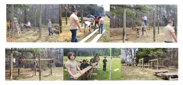
Then it was time to install the roof. I learned how to set the "king posts" that the ends of the main roof beam sit on and then we got to work cutting and installing the 2x6 trusses for the roof. Uncle Ray also donated a recycled metal roof which is better than the wood slats roof I originally planned because it will last longer and it won't have to be repainted every year. After the trusses were set, we installed the perlins for the metal roofing.
