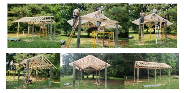
The metal roof and gable were installed with special screws/gaskets so it doesn't leak.
